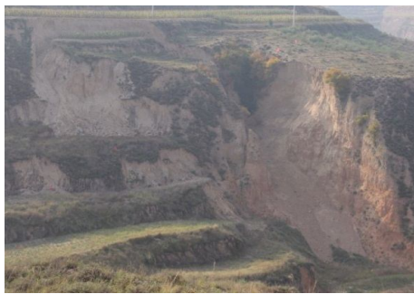
图3 洞外地表坍塌 Fig.3 Surface collapse
